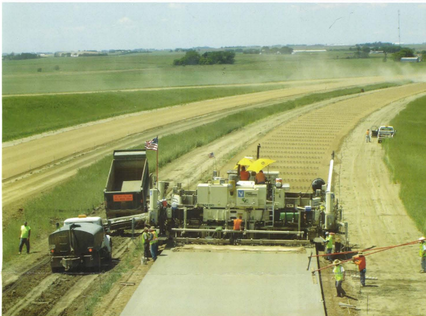
Cedar Valley Corporation paving Highway 60 corridor in Northwest Iowa with G&Z's S850. The mainline paving was done at a width of 25.6' (7.8m) and with varying thicknesses of 10.2" - 10.6" (260mm - 270mm). The five separate projects had similar smoothness averages of 17.4"/mile (280mm/km) on a zero blanking band.
